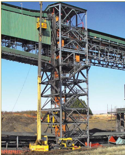
Full view of counter weight installation.
